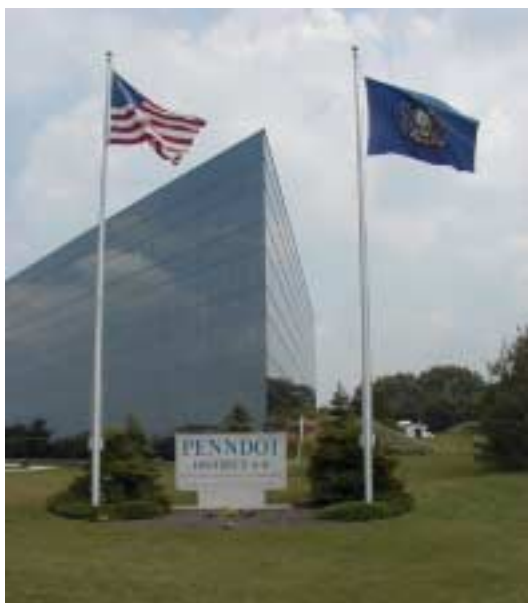
PennDOT's New Headquarters in King of Prussia
